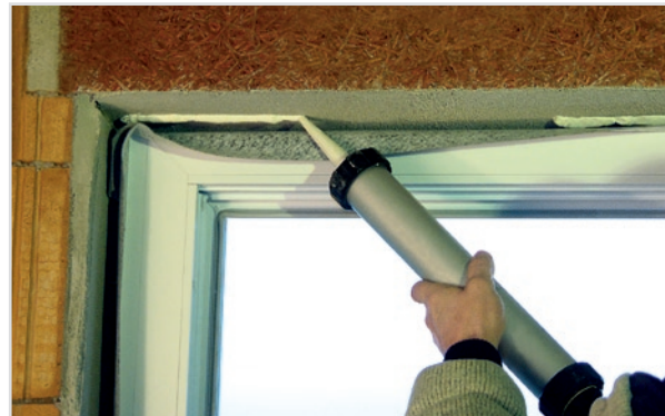
Installation example: iso 3 -Window Sealing System
